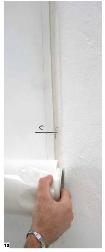
When you have checked that the panel is correctly centered, please fold 10 cm of bisilicon paper (13) and start applying the prints on the free area (14).
