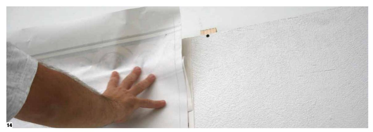
Hold the printed paper away from the wall, get rid of half of the bisilicon paper and continue the application on the rest of the free area (15). Continue with the TATTOO-WALL application pressing the surface of the paper with your hands, from the middle towards the sides to let the air out (16-17).
