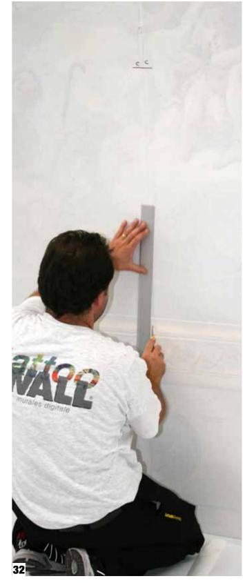
Remove the junction silicon stripe (33-34-35) and press the edges of the panels you have just cut (36-37).
