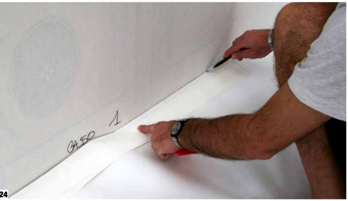
Get ready to place the next panel checking the progressive number and cutting off the first 5 cm of bisilicon paper (25) so that the panel start sticking to the wall. Check the correct positioning in both vertical and horizontal way (26-27).
